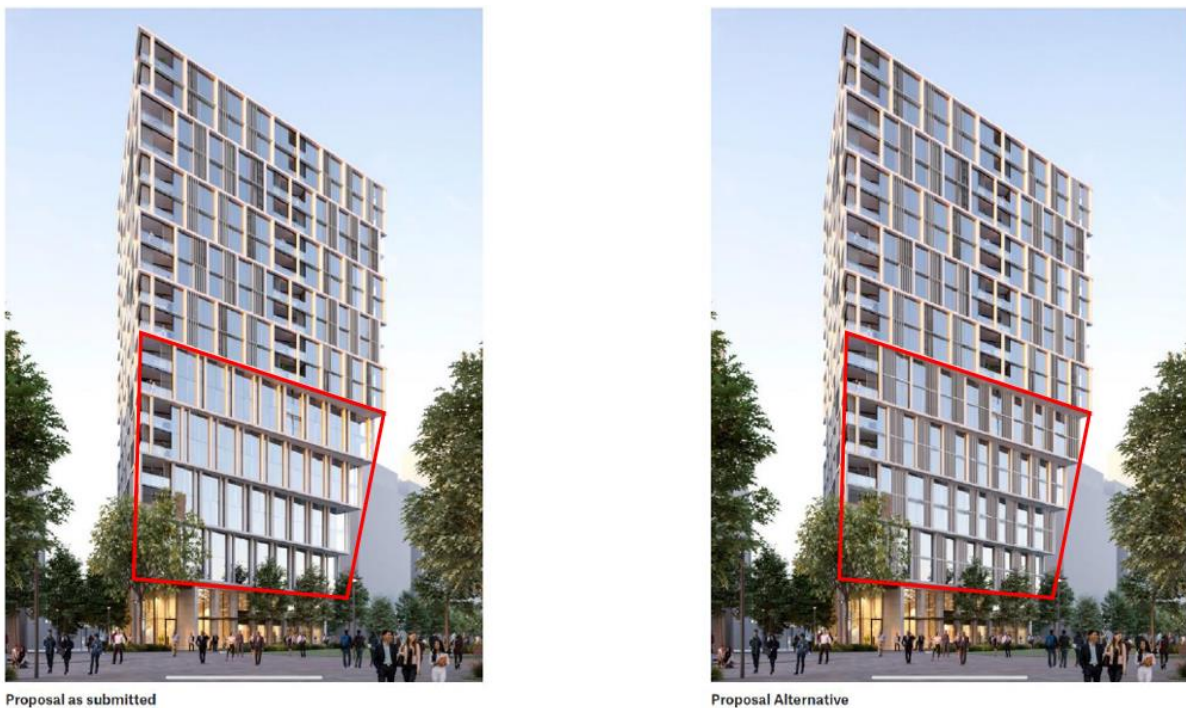
Figure 71: Photomontages comparing the proposal as submitted vs as amended. The external shading has been extended down to the south-western facade within the area outlined in red.
