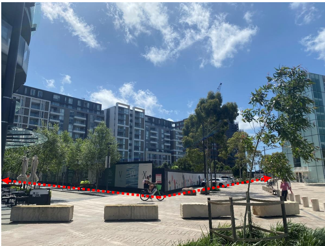
Figure 4: Site viewed from Green Square Plaza at Botany Road, looking east
