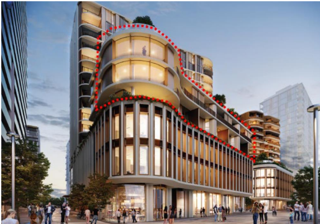
Figure 68: Apartments of concern on Site 7 outlined in red
