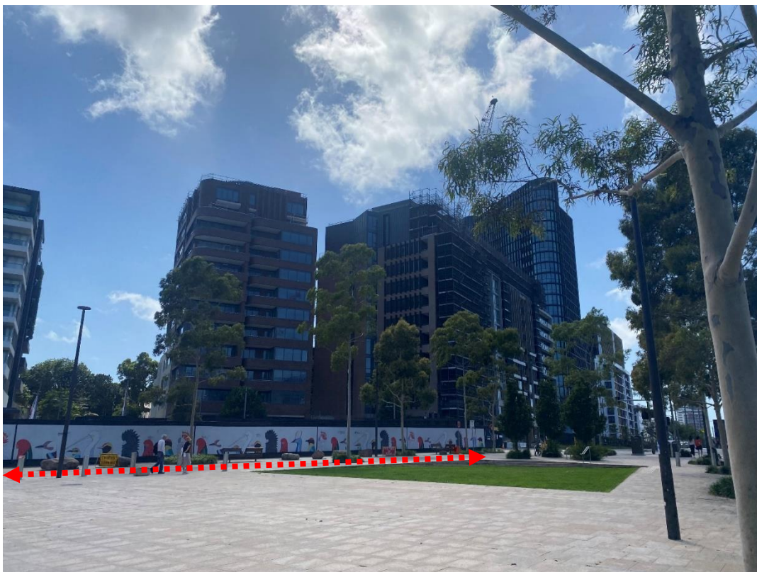
Figure 6: Site viewed from Green Square Plaza, looking north-east towards Site 15
